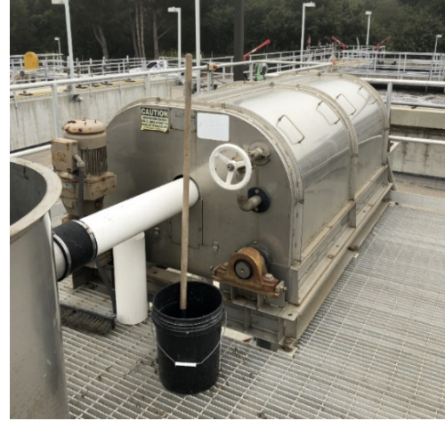
Figure 11: Sludge thickener
