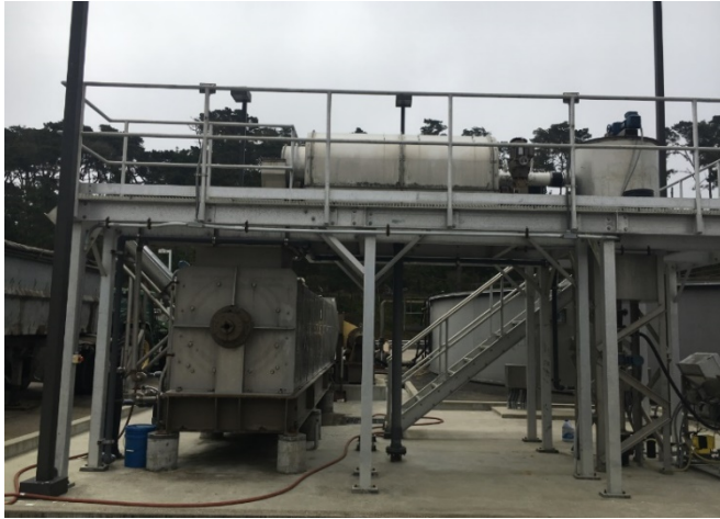
Figure 10: Sludge thickener and screw press
