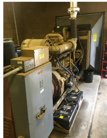
Figure 12: Emergency generator
