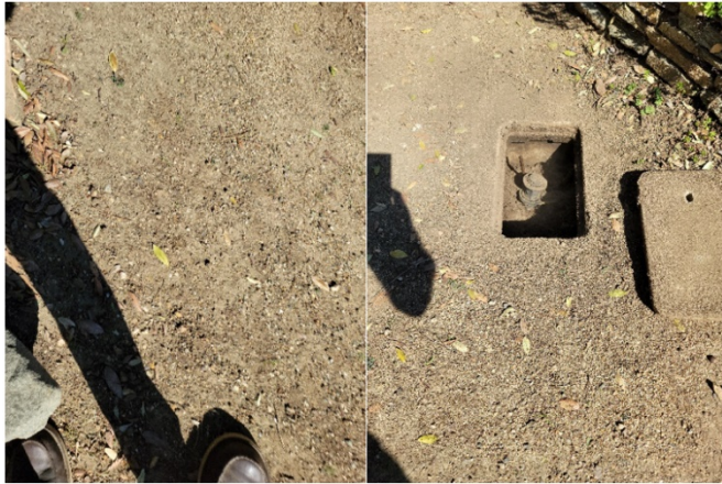
Figure C - Meter location covered by dirt (left); uncovered meter (right). Without locating and documenting the meter location in GIS, finding this meter box would have been very challenging.
