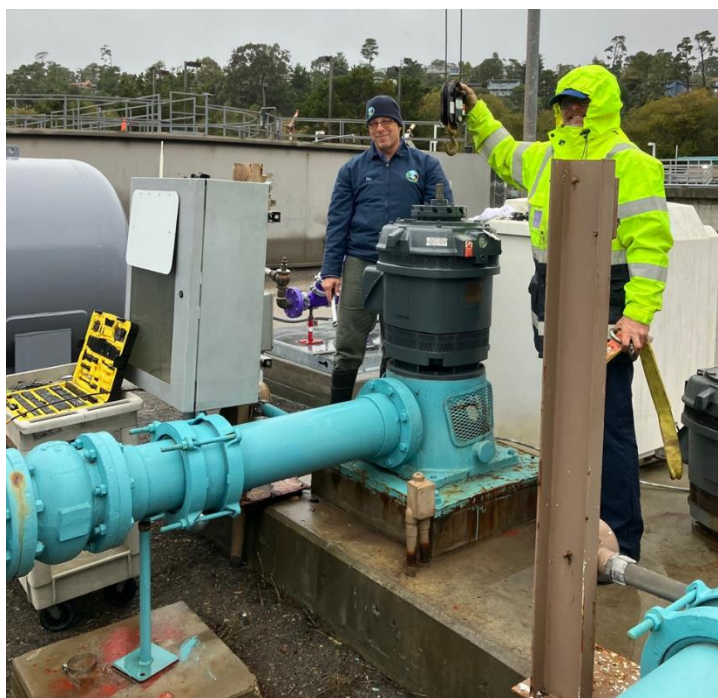
Figure 1 - Effluent Pump Motor #1
