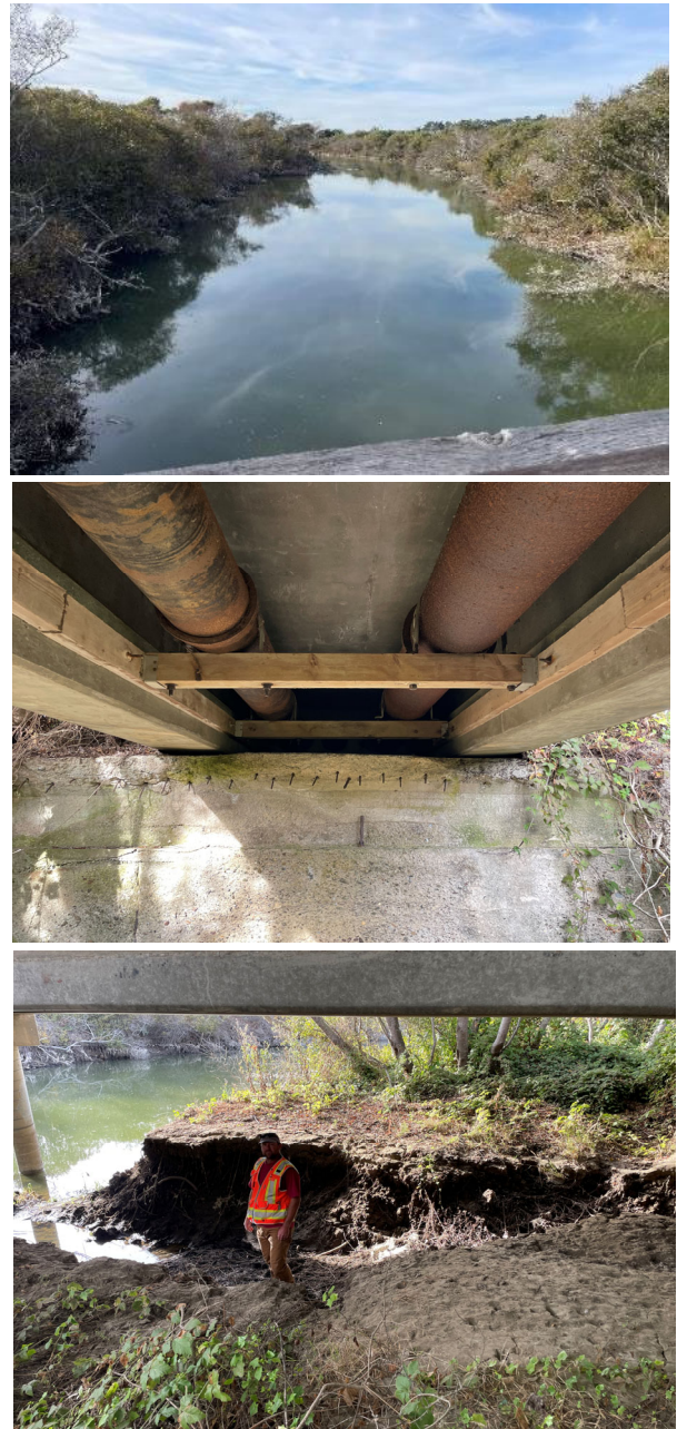
Figure 3: San Simeon Creek Conditions below Bridge on 11/14/23
