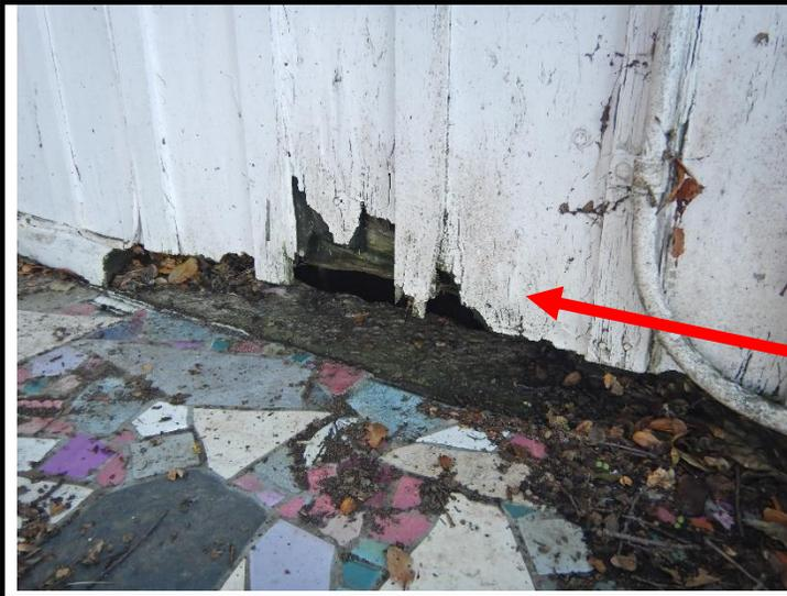
1 **Areas of excessive moisture and / or bug type damage and deterioration found at areas of the structural wood framing.**
