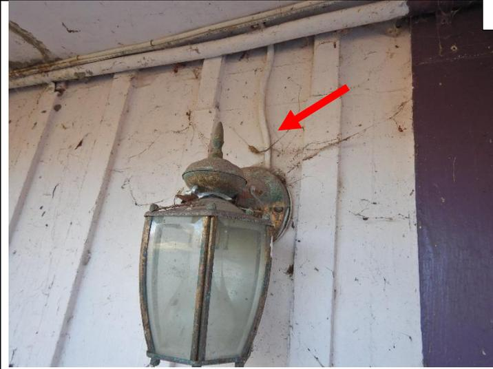
5 **Improper wiring / Exposed electrical wiring or "Romex" found not installed to minimum standards subject to physical damage not in a conduit or raceway per standards. Safety Hazard: ON THE EXTERIOR AT THE FRONT ENTRY LIGHT**
