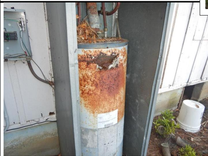
11 **The Water heater is defective, damaged, improperly installed and unsafe.**
