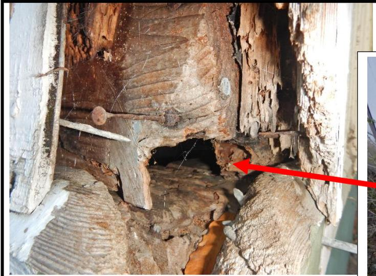
10 **Areas of excessive moisture and / or bug type damage and deterioration found at areas of the structural wood framing.**
