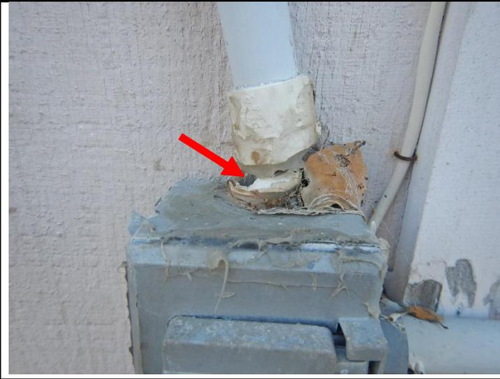
6 **A broken electrical conduit found at an added exterior outlet. Safety Hazard.**
