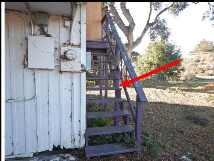
2 **Exterior stairway to the upper living space found improperly constructed and are unsafe. Safety Hazard.**
