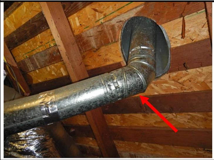
12 **Missing the proper strapping at the furnace vent piping in the attic at the horizontal to vertical transition through the roof**
