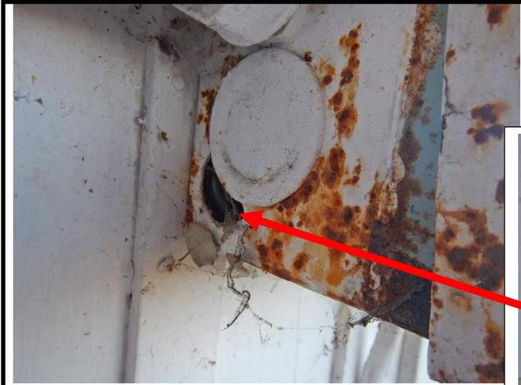
4 **Unprotected / unused opening(s) through the SIDE of the MAIN ELECTRICAL PANEL needing to be sealed for safety per standards. This will help prevent critter intrusion into the electrical panel.**
