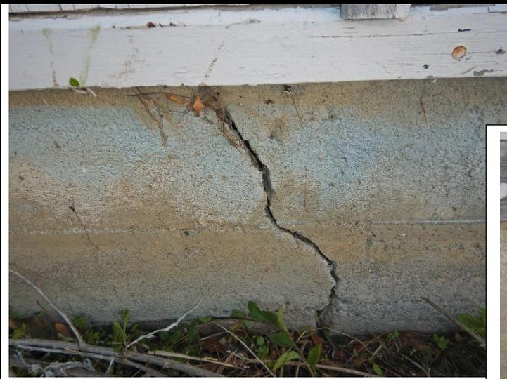
13 **Some moderate cracks and/or displacement of the raised concrete foundation perimeter stem wall noted in multiple areas. This may be indicative of unusual settling or movement of the soil around the foundation.**
