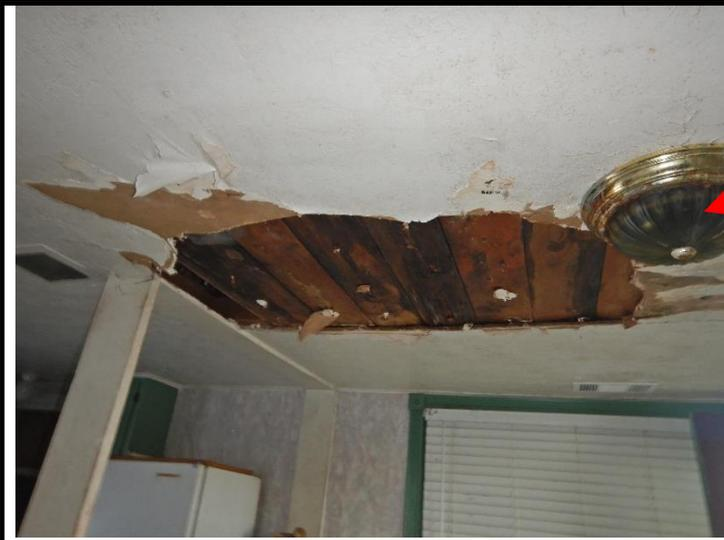
16 **Heavy active water leaking and damage found in areas of the interior ceilings / wet today. Evidence of mold.**
