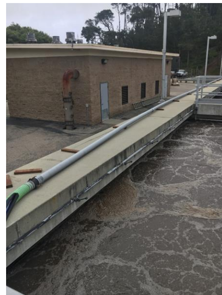
Figure 8: Aeration Basin and Blower Building
