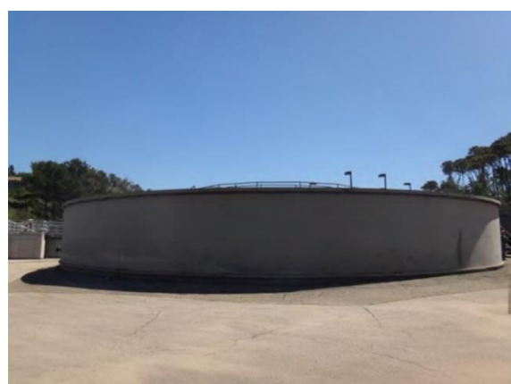
Figure 5: Existing South Clarifier (from west)
