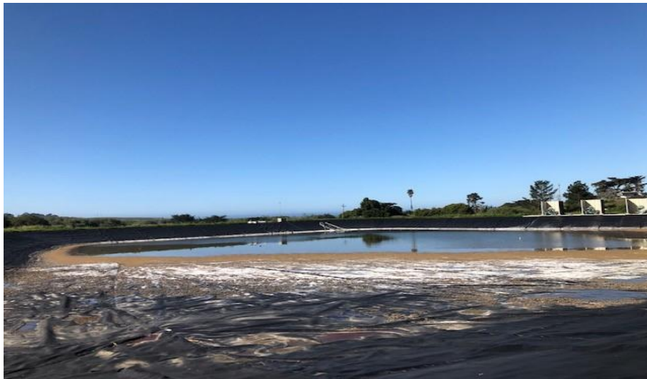
View of Brine Pond from North East taken April 17th.
