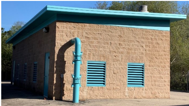
Figure A Freshly painted building at the WWTP.
