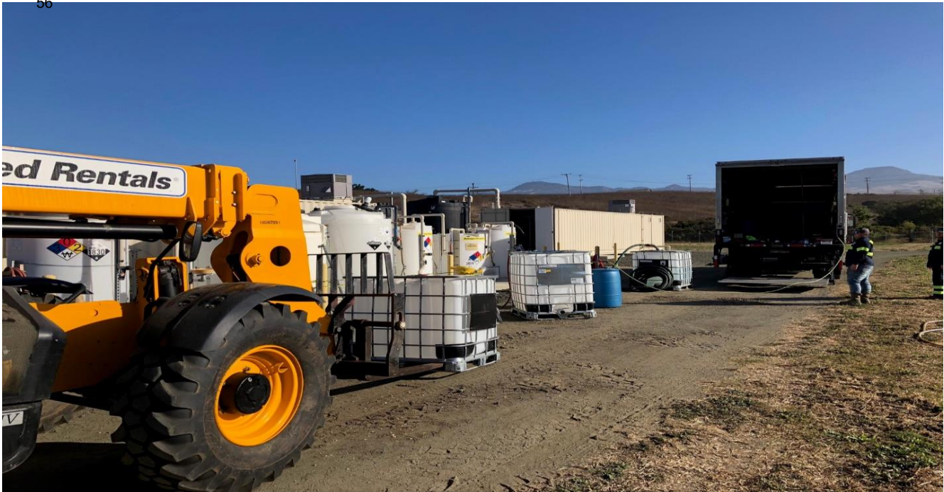
Photo of Recent Work by Chemical Supplier Brenntag in Replacing the Sodium Hypochlorite tank, which had a bad fitting.
