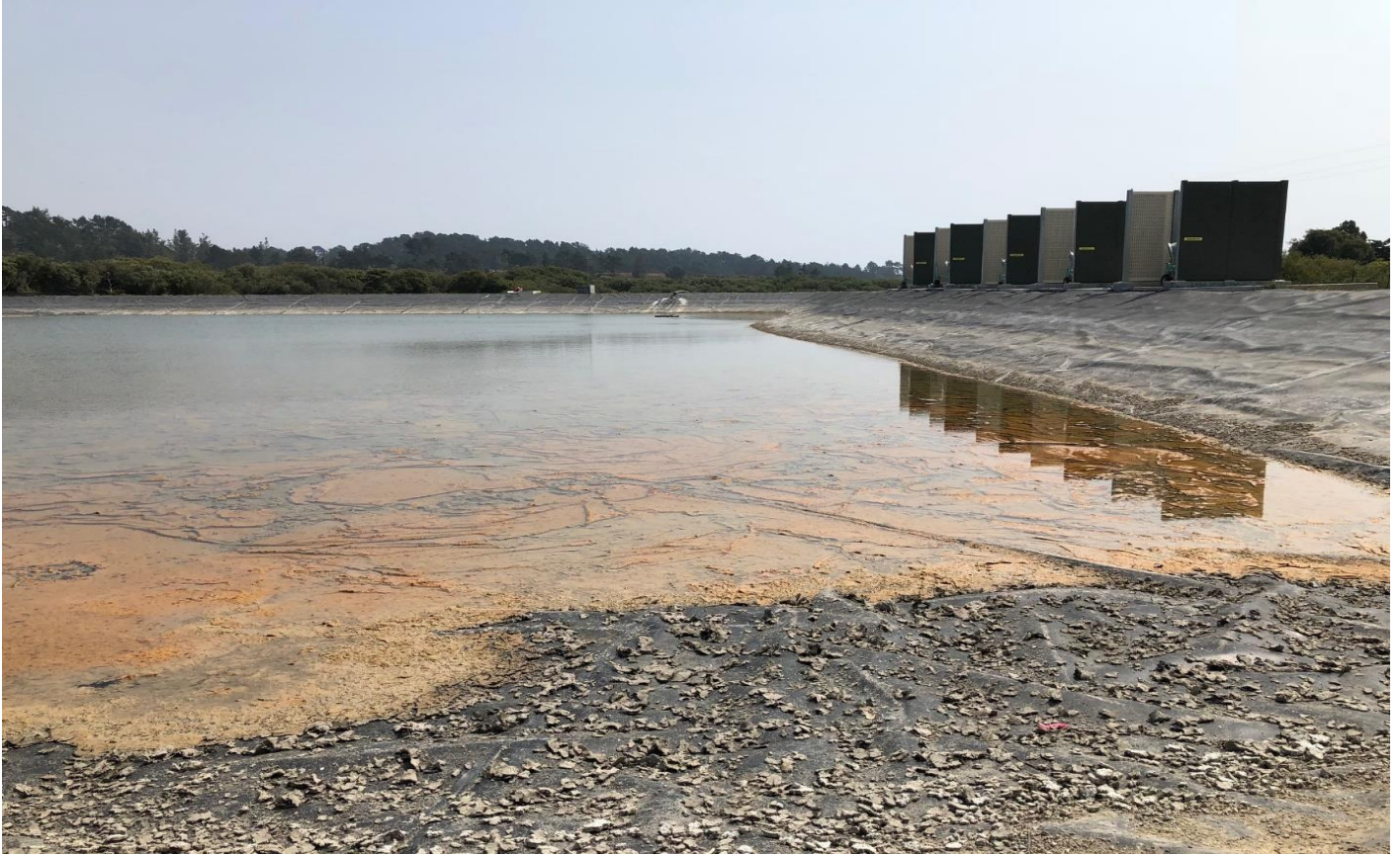
Photo of impoundment basin on August 30, 2018 from its northwestern corner looking south. Beyond our work on the SWF, we continue to assist the Water Department on leak repairs and in other areas as needed.
