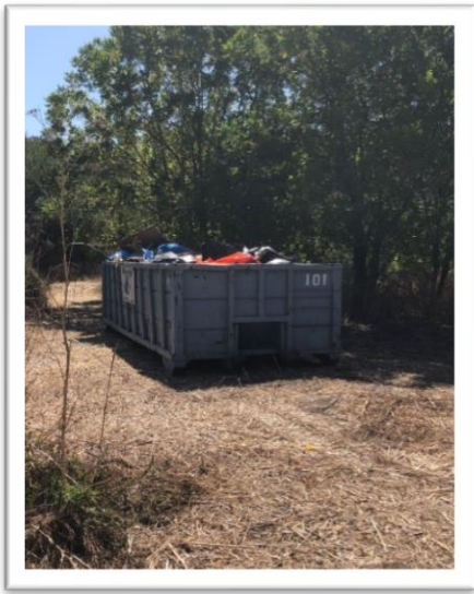
Figure 9: 20cy roll-off, filled within 6 hours of delivery to the site.
