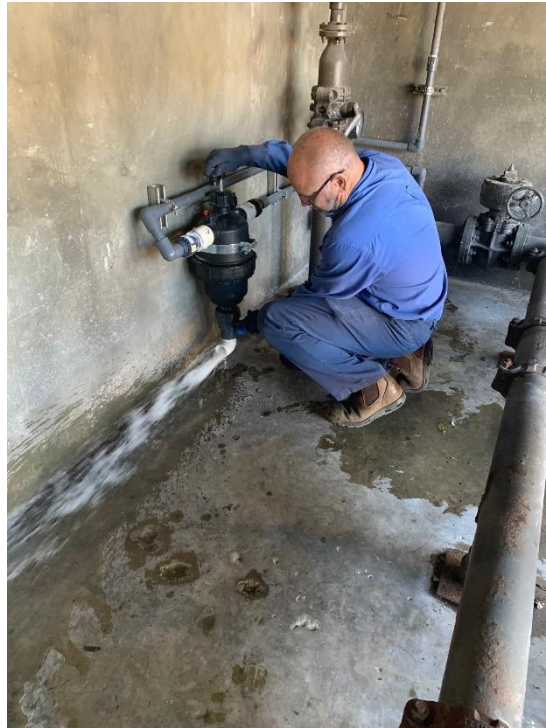
Figure B - Toni Artho installs new filters at the WWTP
