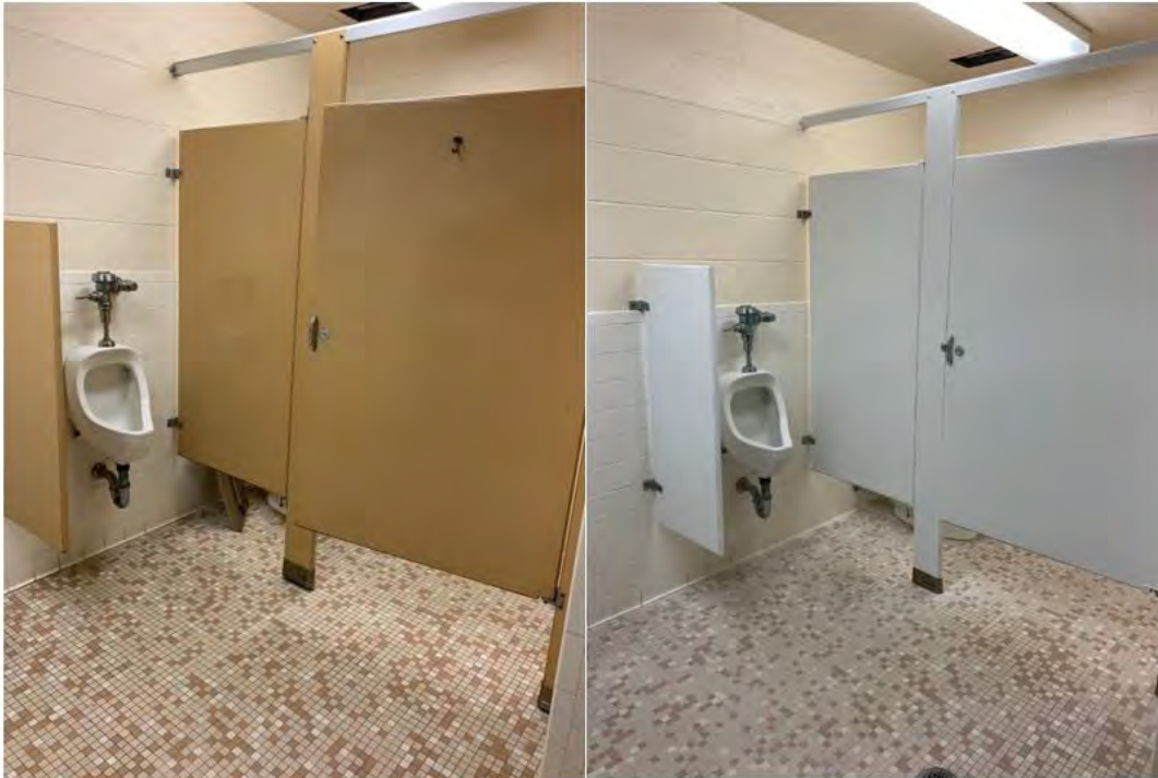
Figure 2 WWTP bathroom before (left) and after (right)
