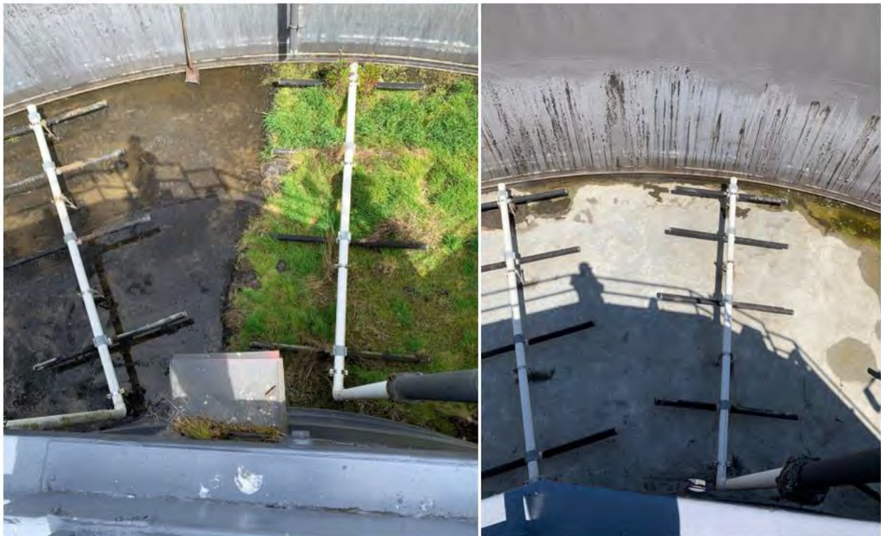
Figure 1 Digester basins before (left) and after (right) test preparations
