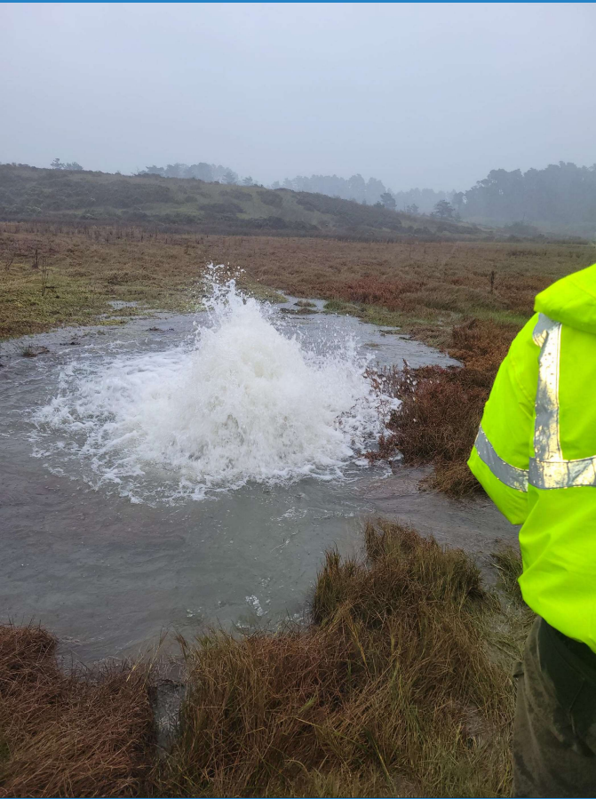
Figure 1- Site location of water main break and proposed repair
