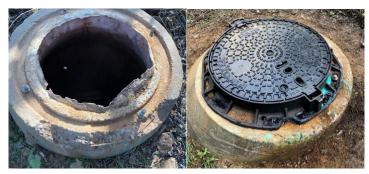
Figure 3 Rehabilitated Manhole
