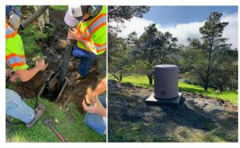
Figure 5 Water operators repairing the failed Air-Vac (left); newly installed Air-Vac (right)
