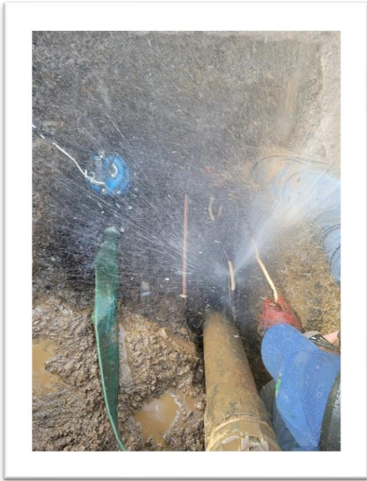
Pictured Left: ¾" Service line 3' below the surface leaking at 3 GPM
