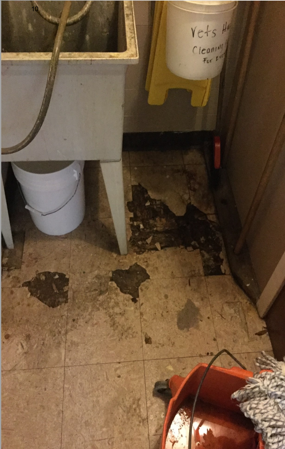
Rotted Floor and Plywood
