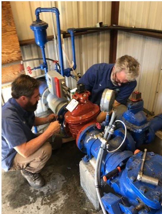
Figure 1 Water staff Lyman and Grosskruetz installing new 6" gate valve.
