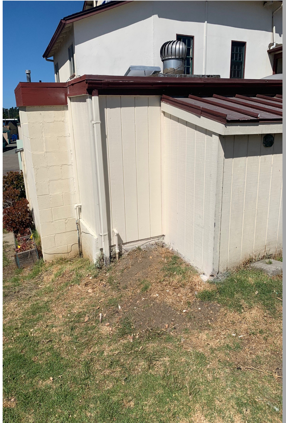
New Siding and Paint
