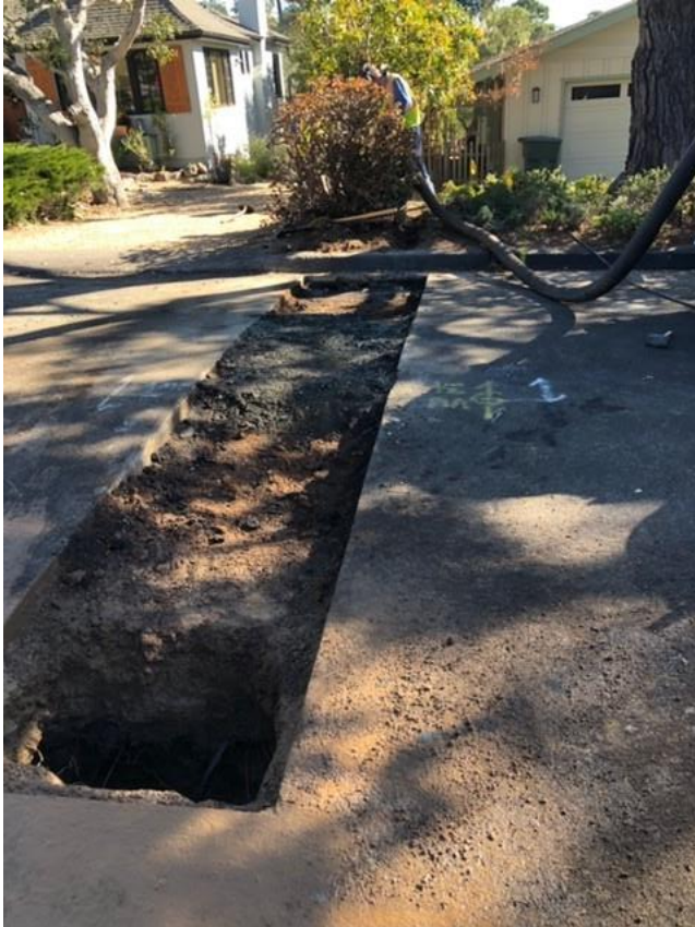
Figure 4 Initial Excavation at Hillcrest Drive
