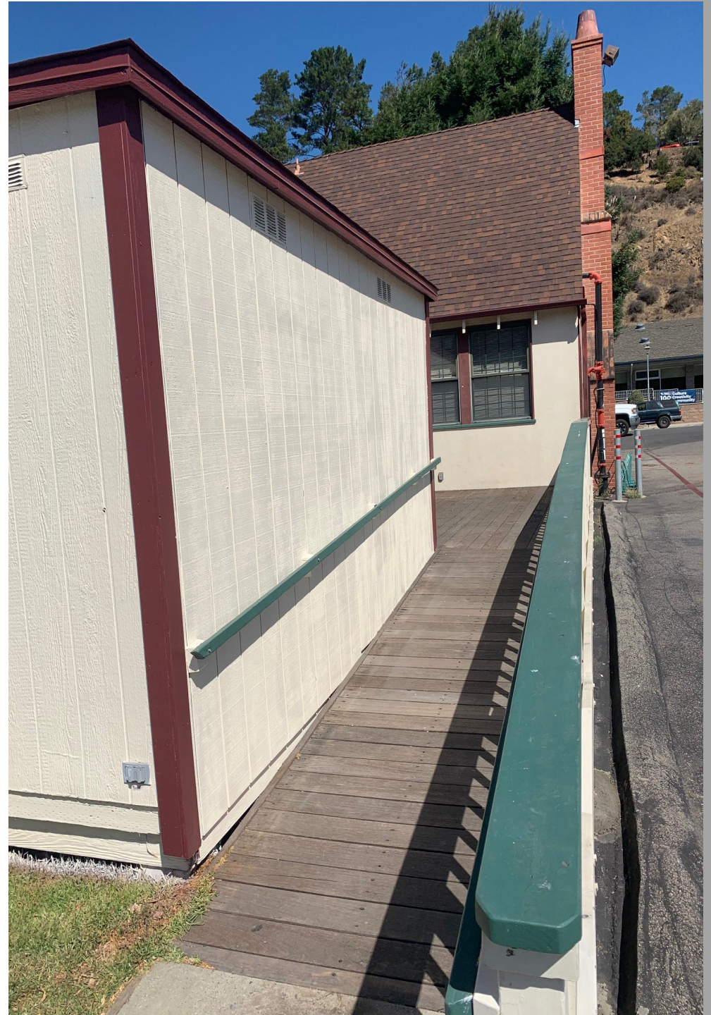
New Roof, Fascia, Trim, Siding, Vents and Paint
