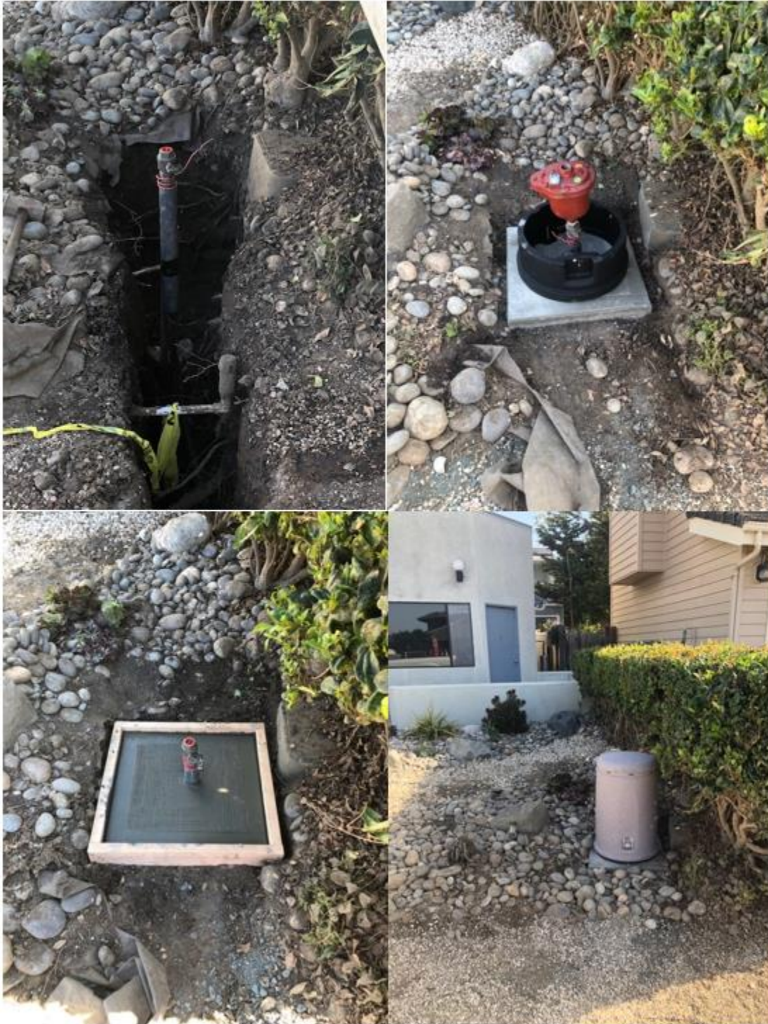
Figure 3 Phases of air vac replacement
