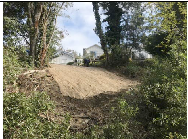
Repair site post seeding and jute netting installation.
