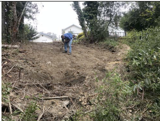
Preparing the site for seeding and erosion controls.
