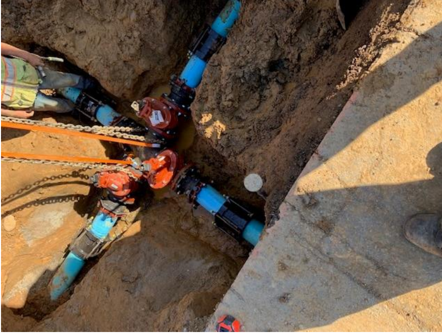
Figure 2 New cross and valve installation at Trenton/Kenneth
