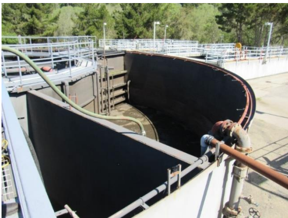
Figure 4: Existing South Clarifier (from south)
