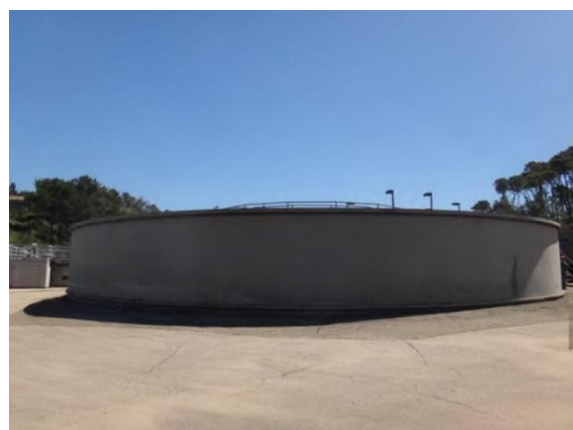
Figure 5: Existing South Clarifier (from west)
