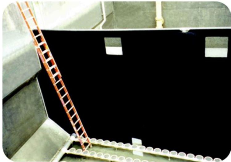
Figure 10: Geomembrane Baffle with Flow-Through Window ( Environetics Director II )
