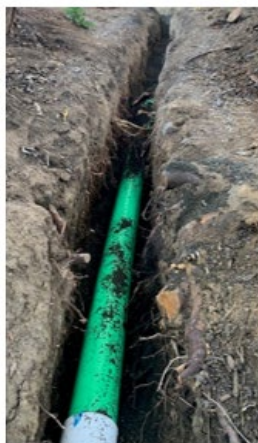
Figure A - Line Repair at WWTP
