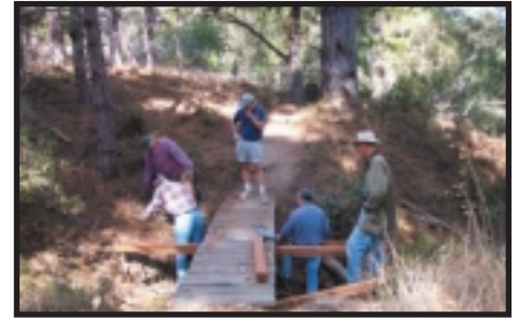
Ranch Hands volunteers repair bluff trail boardwalk.
