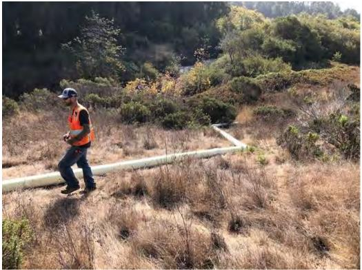
During the month of November, the 8-inch reinjection line, which carries treated water from the Advanced Water Treatment Plant to the reinjection well approximately 1800 feet away, was relocated. Erosion of the cliffside along a stretch of San Simeon Creek had placed the line in danger. Several 45-degree elbows and 50 feet of additional piping were installed to reposition the line further up the hill.
