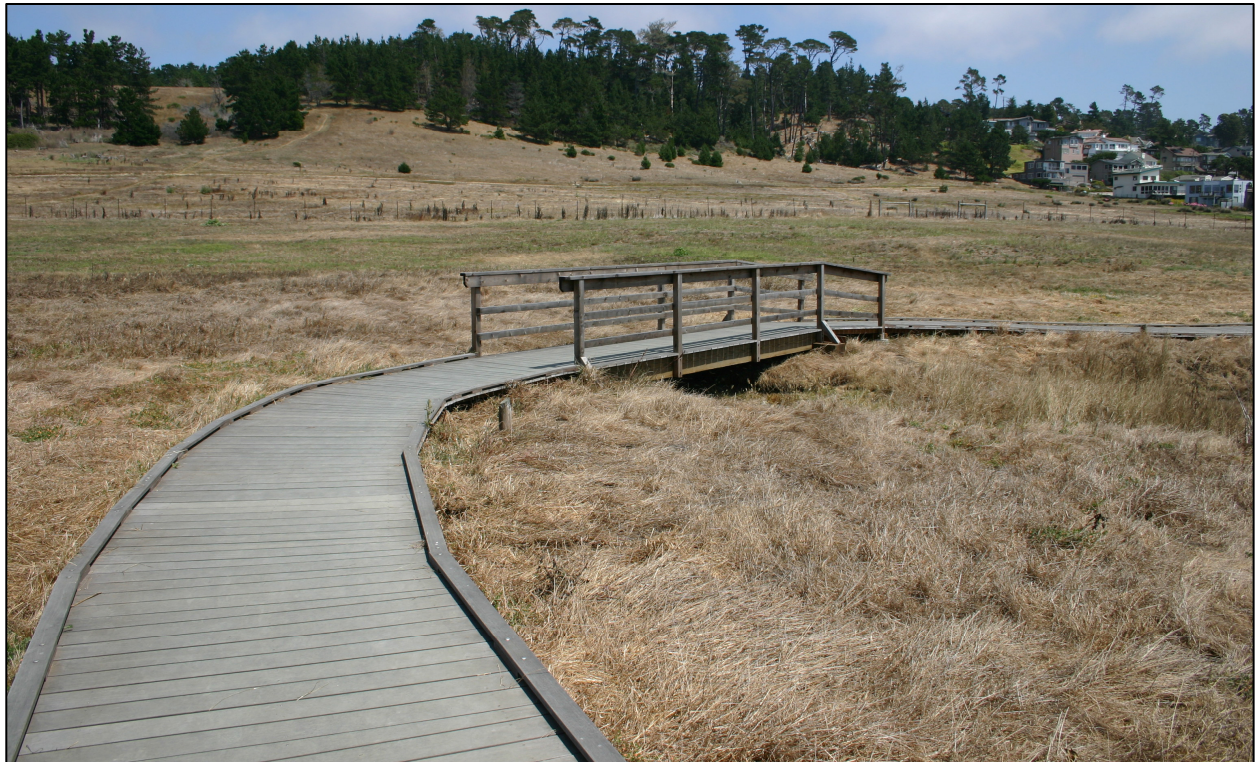
Existing Bluff Trail Improvements FIGURE V-23
