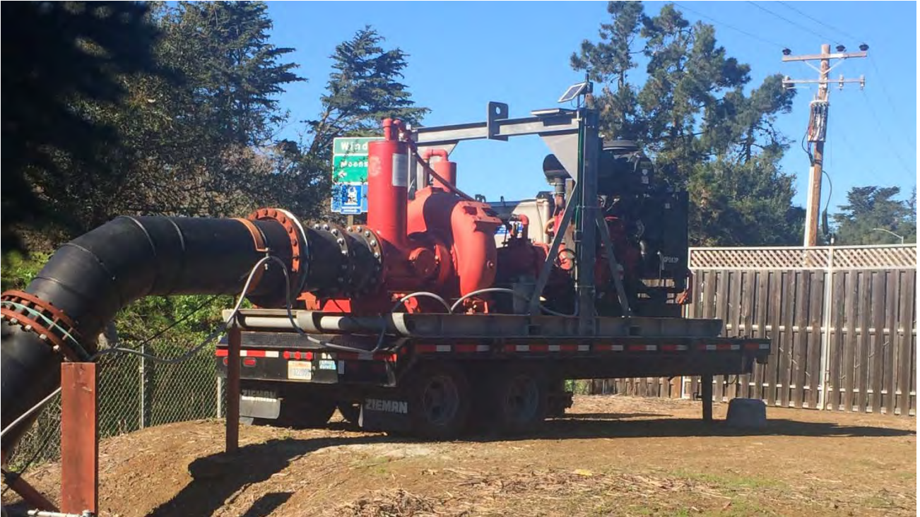
Flood Pump on Main Street - West Village
