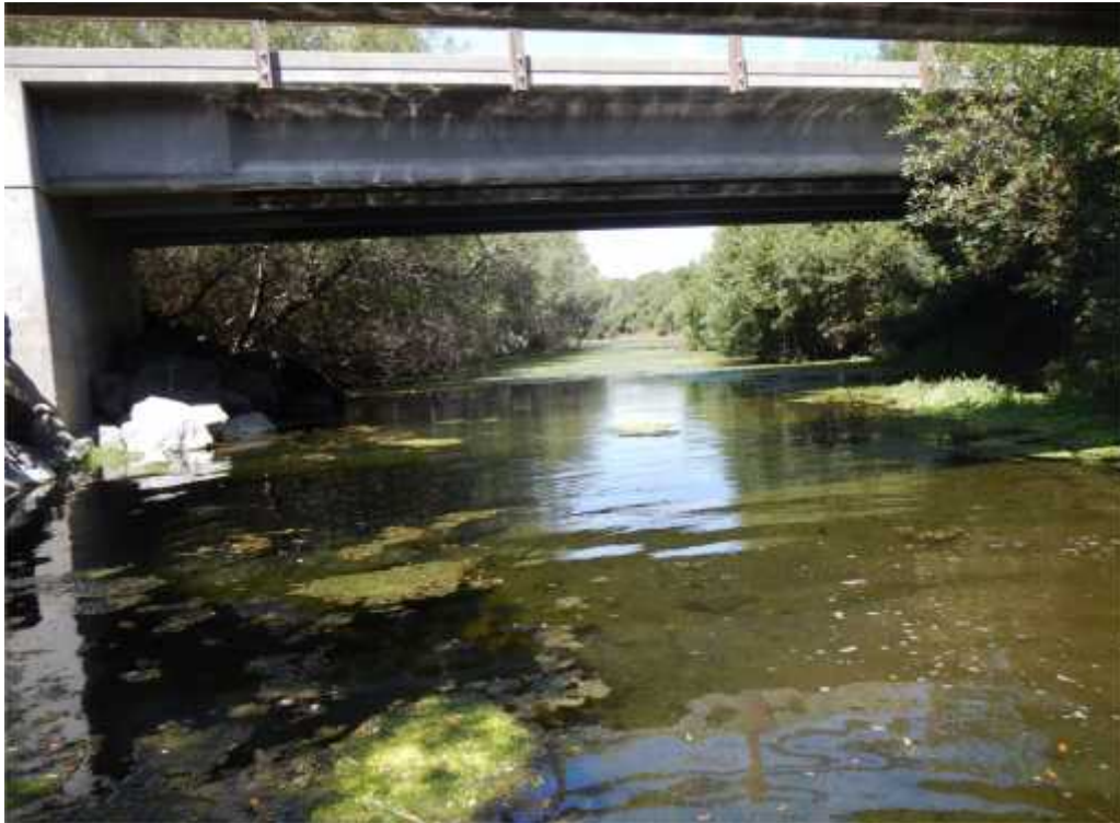
Photograph 13 – View looking northwest of San Simeon Creek flowing underneath Van Gordon Creek Road in the western portion of the project site.
