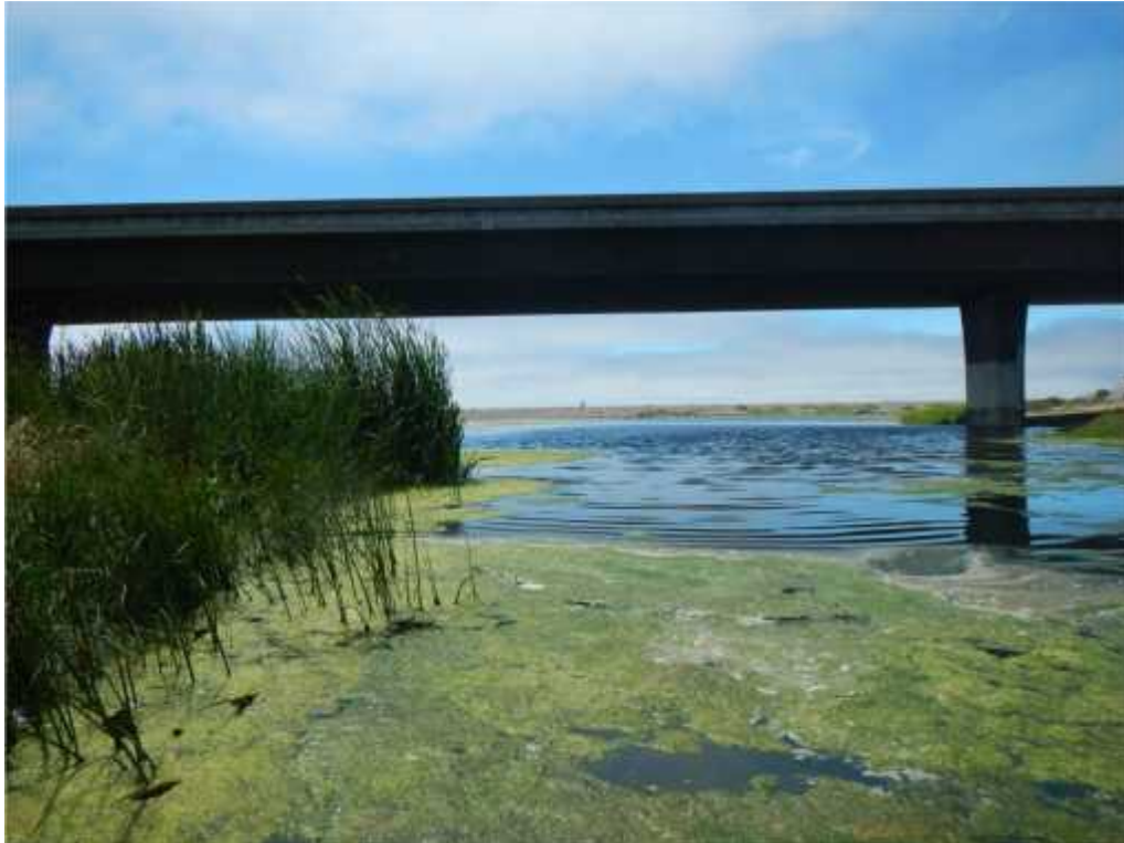
Photograph 16 – View looking southwest of San Simeon Creek and Highway 1 near the western boundary of the project site.
