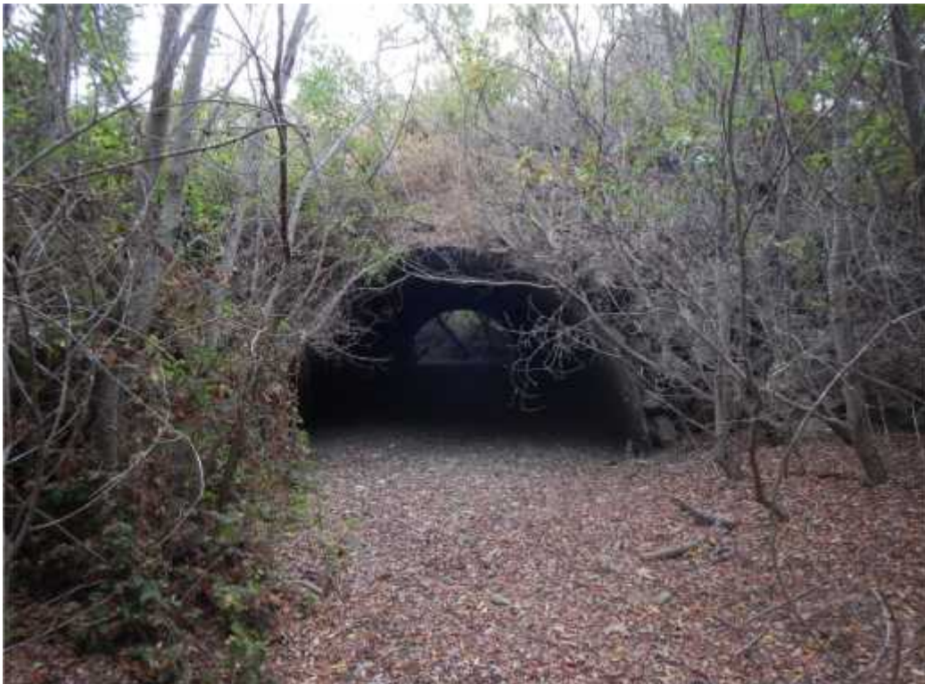
Photograph 18 – View looking northeast of 15' corrugated metal pipe culvert and Van Gordon Creek in the northern portion of project site.
