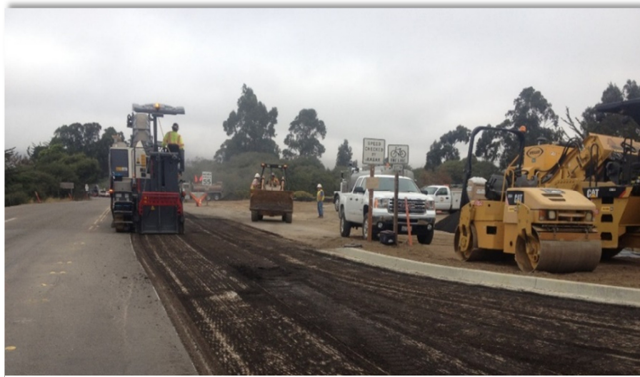
South Bay Boulevard Pavement Grinding
