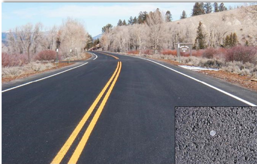
Hot Asphalt Concrete Pavement
