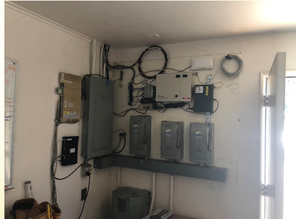
This is after the old wiring was removed.
