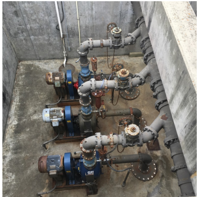
Figure 4: Influent pump station
