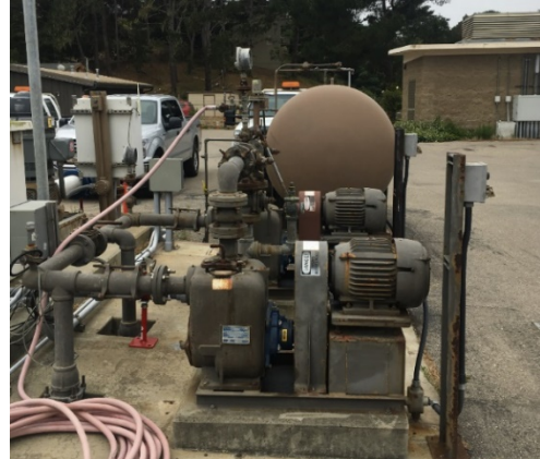
Figure 13: Secondary water pump station
