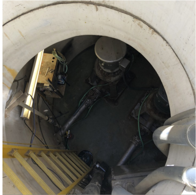
Figure 16: Lift station B4
