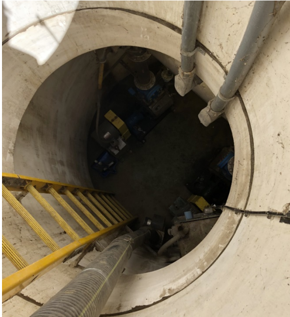
Figure 15: Lift station B1
