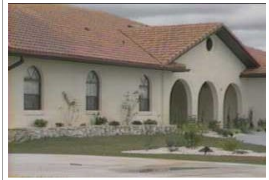
Photograph 11.3. Noncombustible Roof
