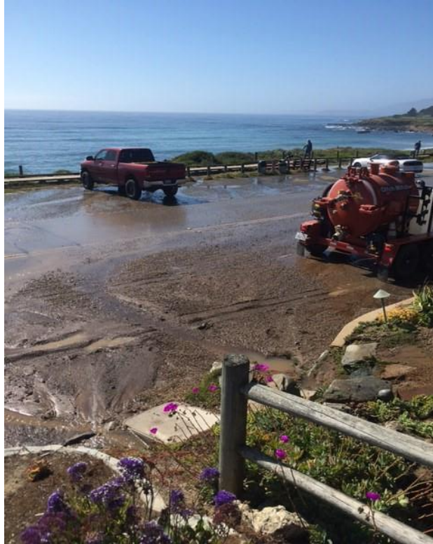
Moonstone Beach Drive leak on April 24, 2019
