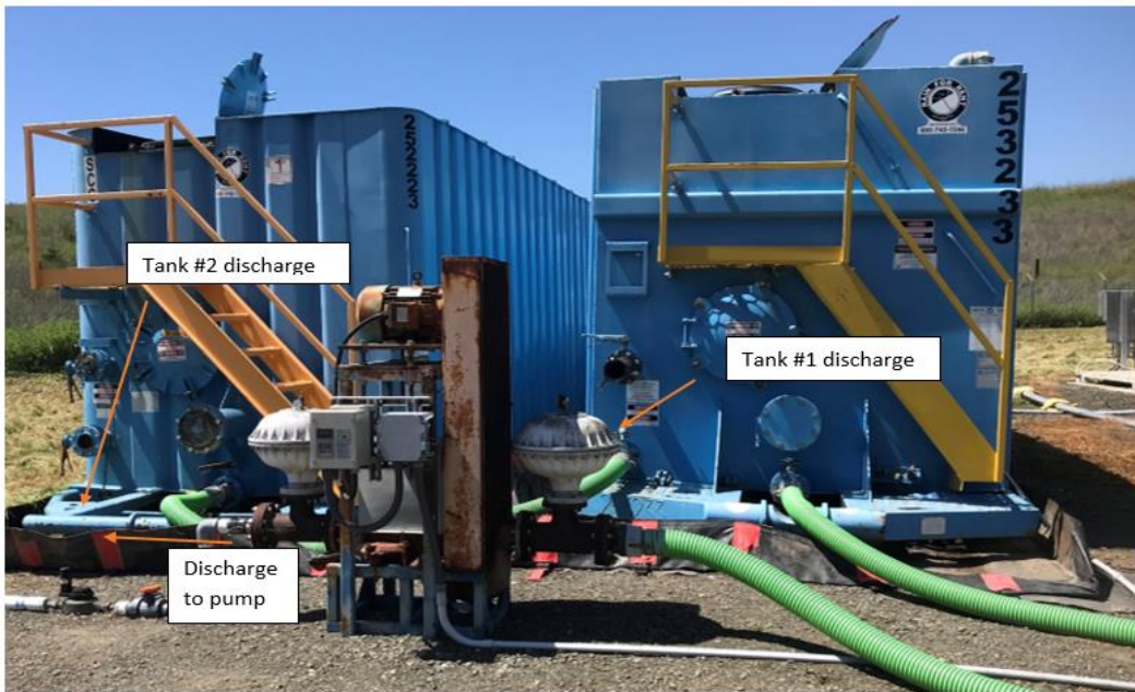
Tank effluent plumbing retrofit for closure plan.
