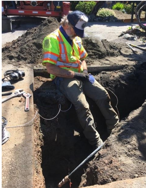
Operator Ben Grosskruetz installing new service and tracer wire.
