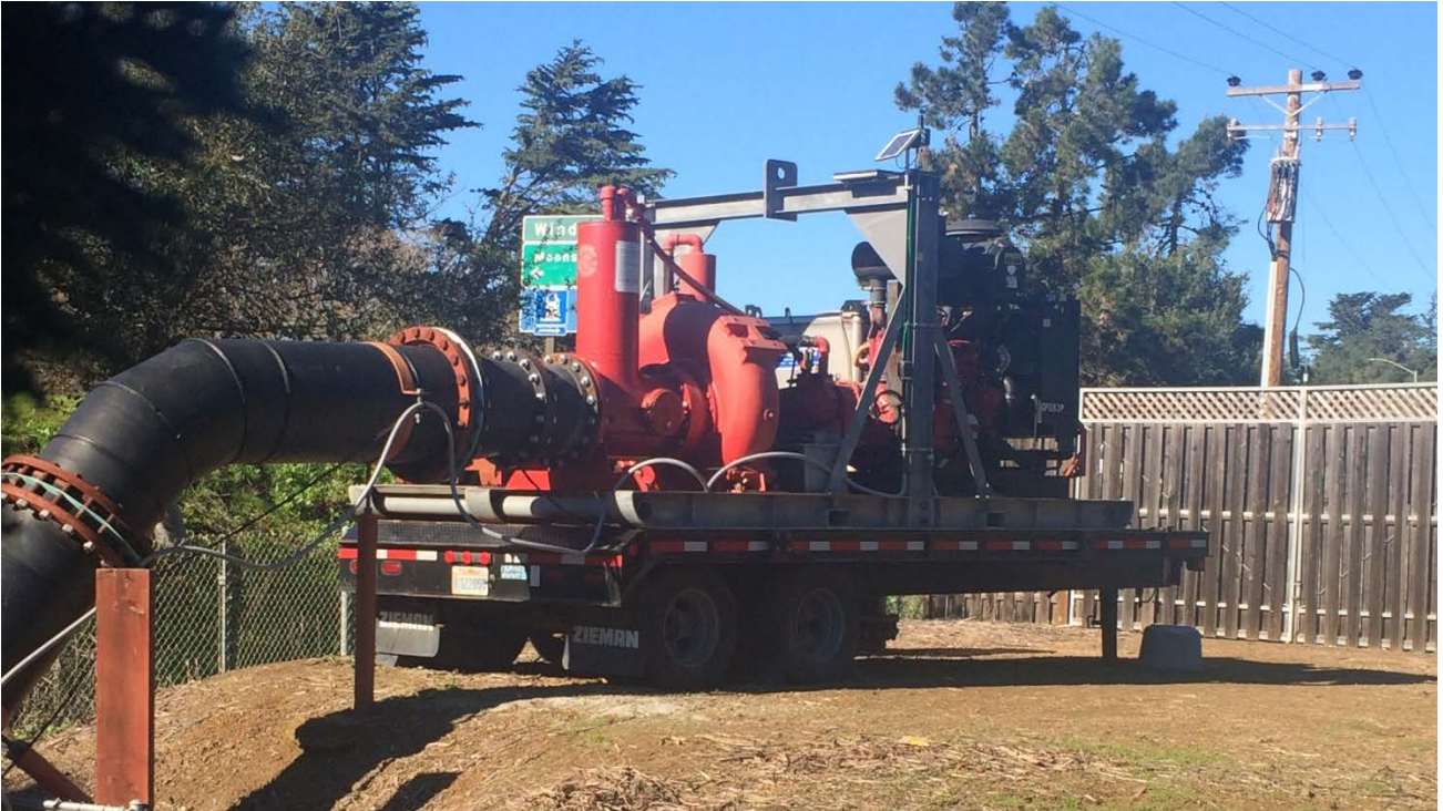
Flood Pump on Main Street - West Village
