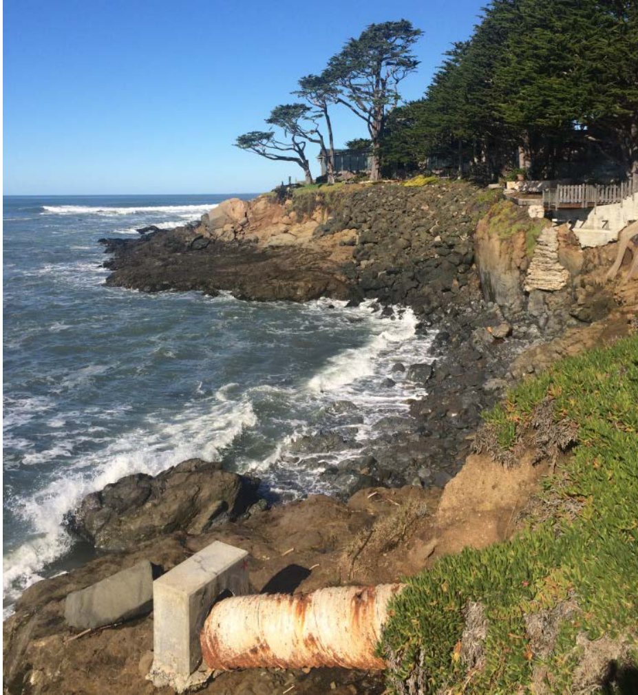
Residential Structures in Tsunami Risk Area
