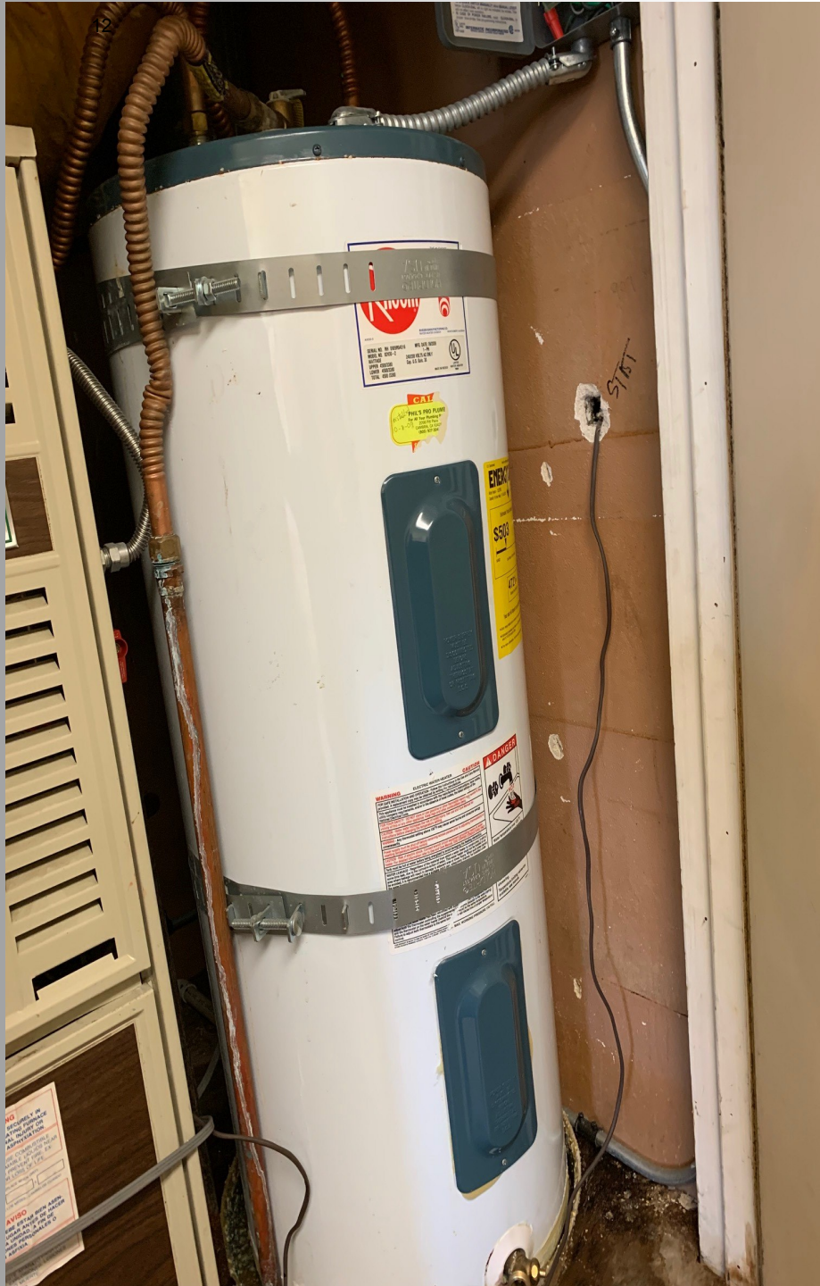
Old Water Heater for Kitchen
