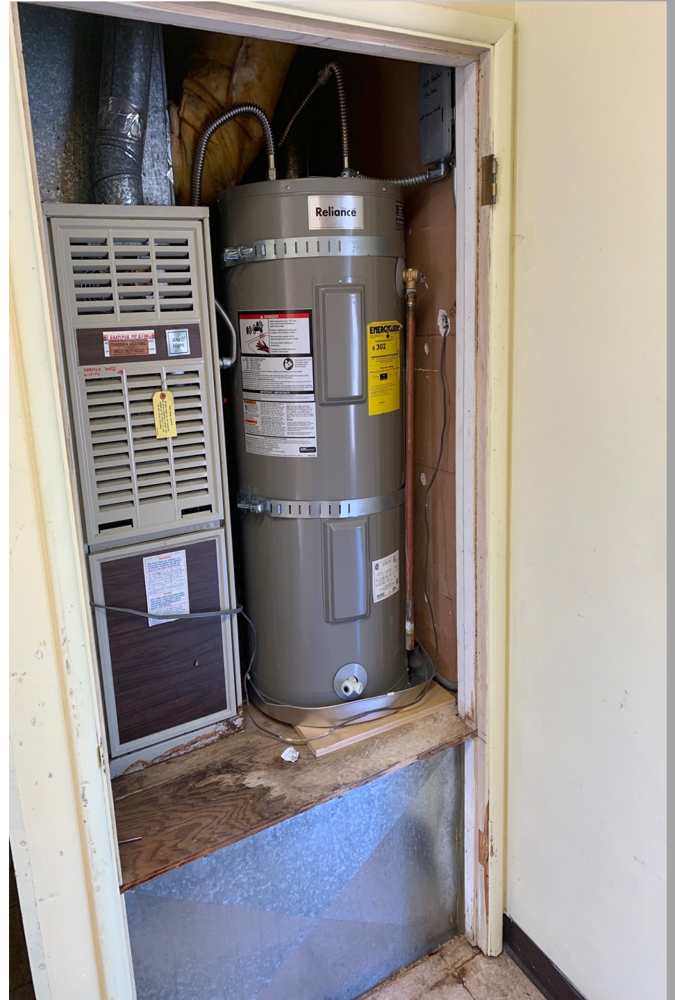
New Water Heater
