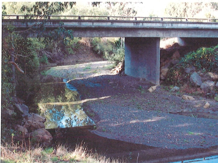
Highway 1 bridge over Santa Rosa Creek
