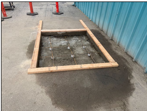
Figure 1: Excavated with rebar added and prepped
