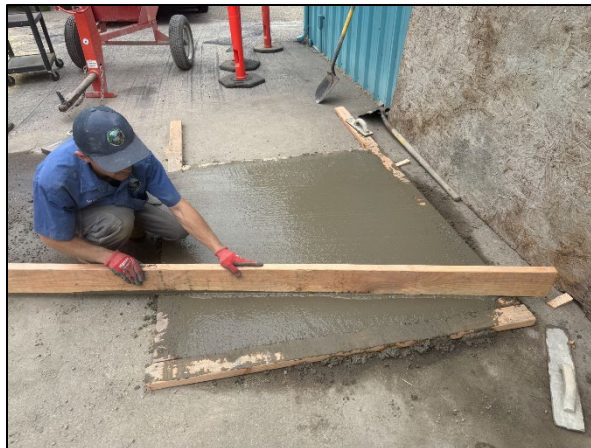
Figure 2: New concrete smoothing
