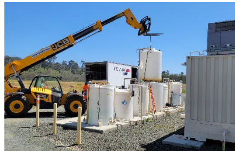
Figure E - Chemical tank retrofit in progress
