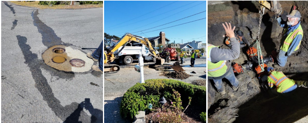
Figure C - Initial leak (left), excavation (middle), and installation (right)
