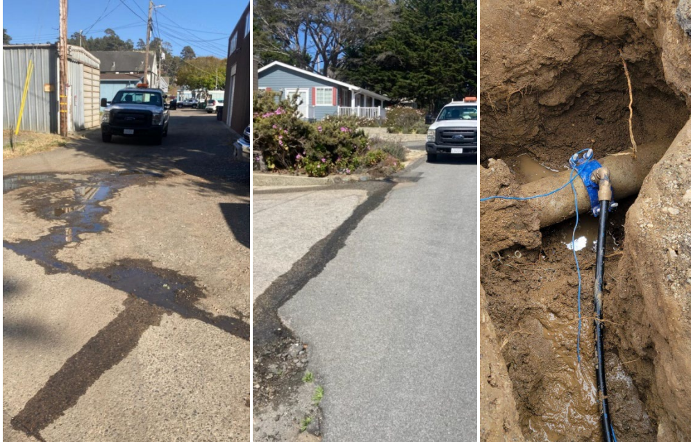
Figure D - Several leaks required attention in May
