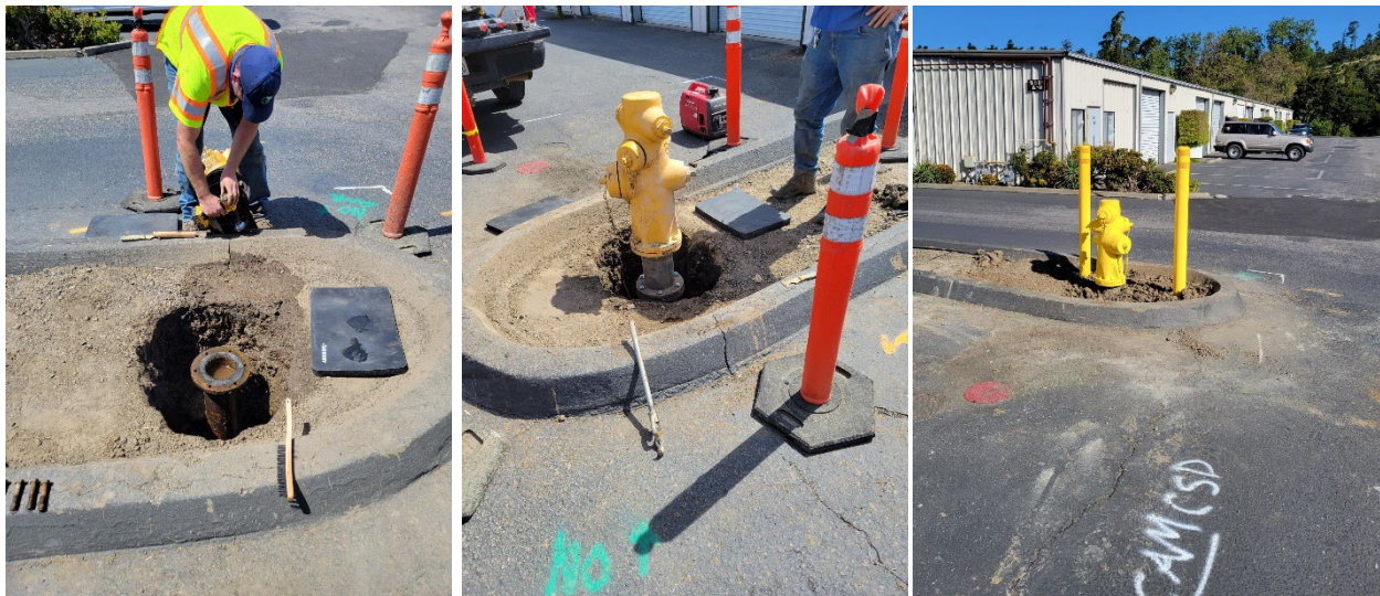
Figure B - Staff preparing the flanged surface for mounting (left), installed and pressure tested (middle), and installed, painted, and protected (right)
