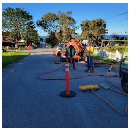
Figure D - Staff busy replacing service lines
