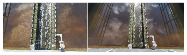
Figure A- Clarifier before (left) and after (right) polymer additive
