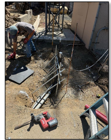
Figure 1: Removal of existing generator, demolition of existing concrete pad, running conduit for new pad & generator.
