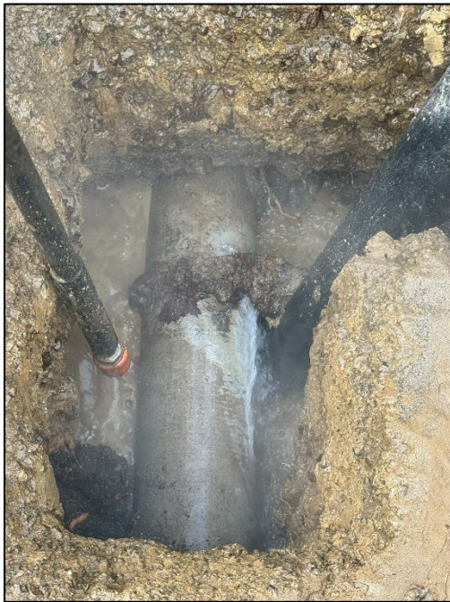
Figure 2: Hudson Avenue leak excavation and repair
