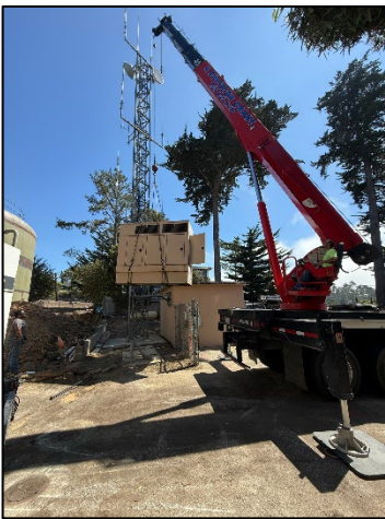
Figure 1: Removal of existing generator, demolition of existing concrete pad, running conduit for new pad & generator.
