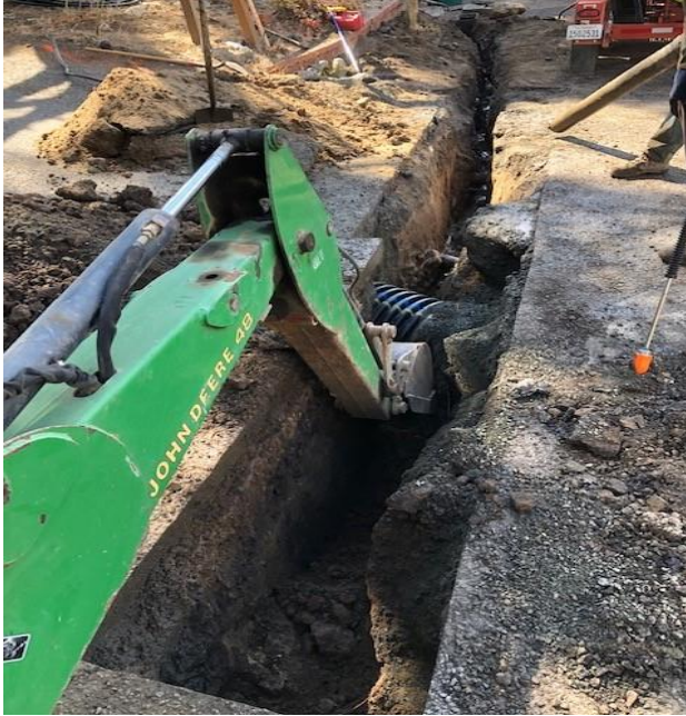
Figure 1 Hillcrest line replacement
