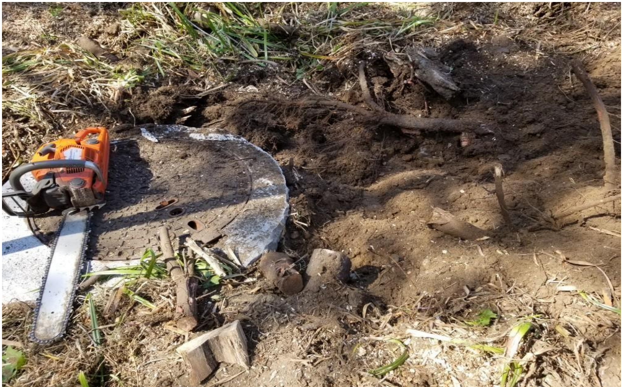
Figure 3 Manhole repair due to root intrusion
