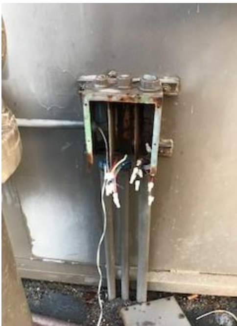
Figure 2 Rusted electrical pull box at digester
