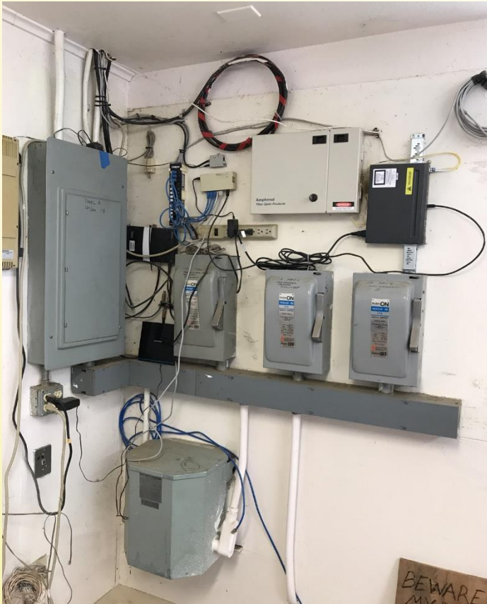
This is before the old wiring was removed.
