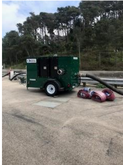
Figure 1 New 6-inch pump
