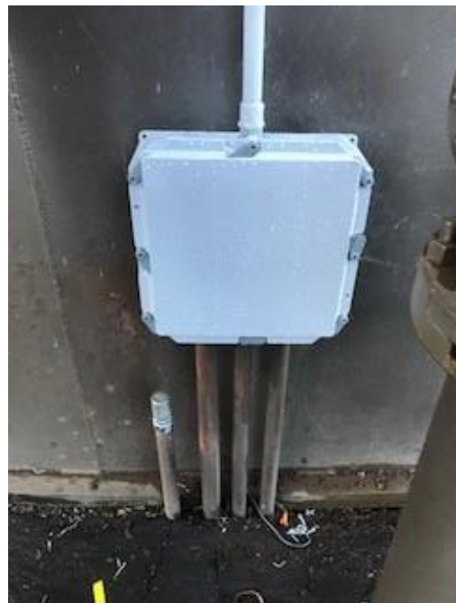
Figure 3 Replacement electrical pull box
