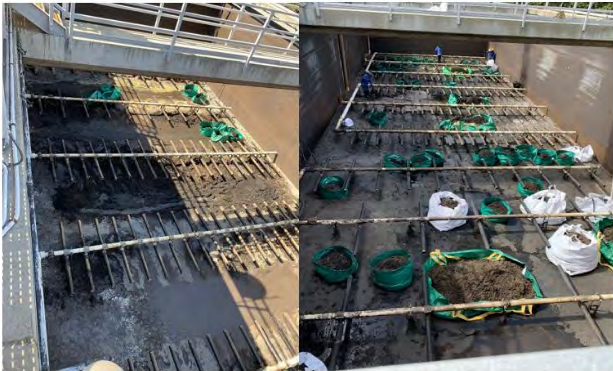
Figure 1 Aeration basin #2 drained and being cleaned
