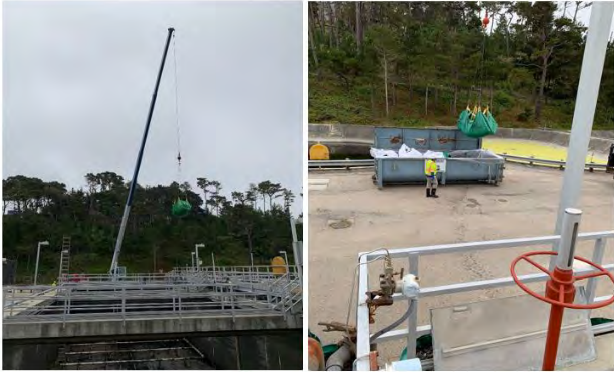
Figure 2 Removing debris via crane
