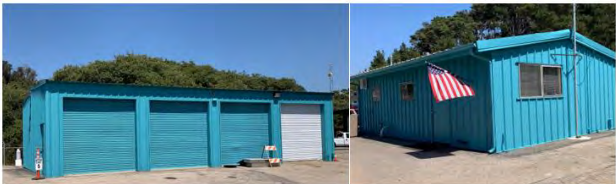
Figure 3 Shop and breakroom with fresh paint.
