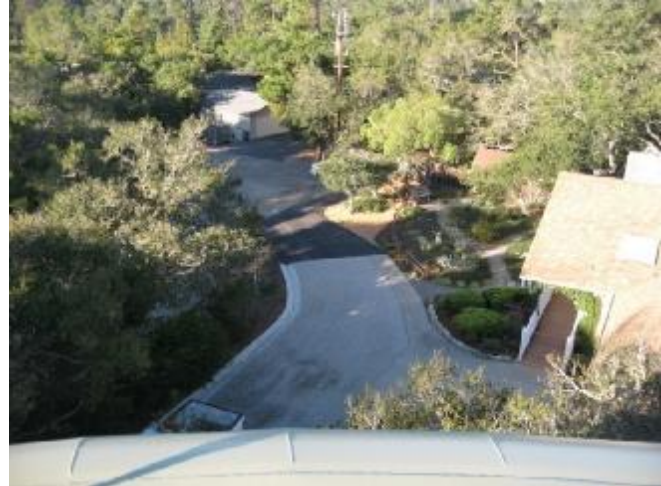
View from top of tank driveway and road repairs
