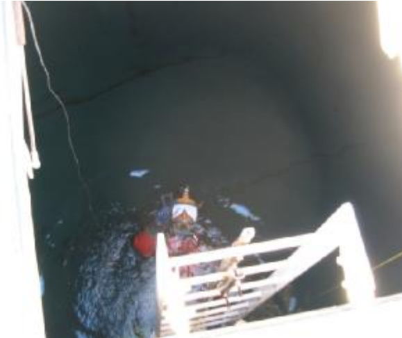
Diver inspecting tank for coating defects
