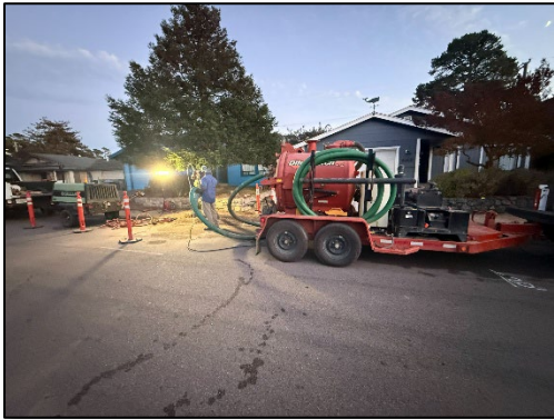
Figure 10: Weymouth excavation prep
