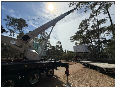
Figure 6: Generator lift for Leimert
