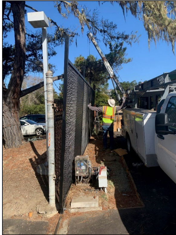
Figure 1: Replacement gate installation at WWTP
