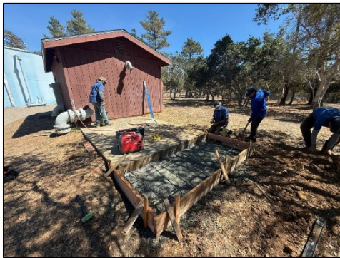
Figure 4: Forms for new concrete in Leimert
