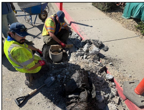
Figure 8: Repairs on Schoolhouse Lane
