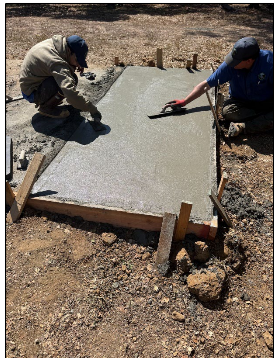
Figure 5: New concrete base for generator replacement
