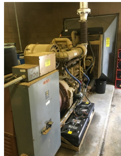
Figure 12: Emergency generator
