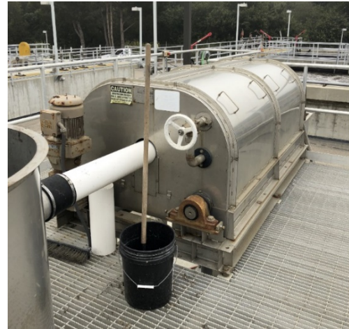
Figure 11: Sludge thickener
