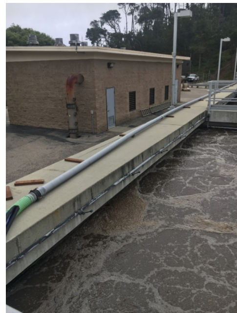
Figure 5: Aeration basin and blower building
