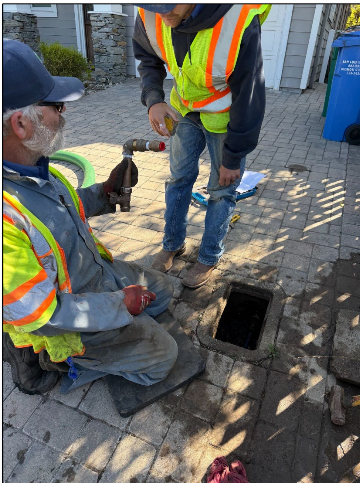
Figure 13: Replacement angle stop
