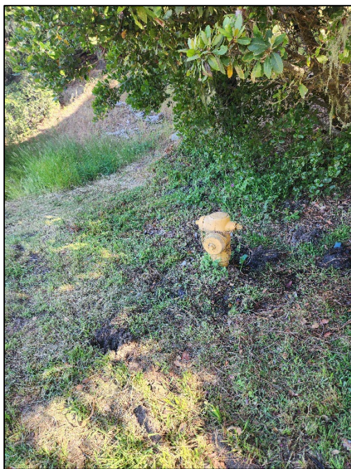
Figure 18: Hydrant before replacement and raising
