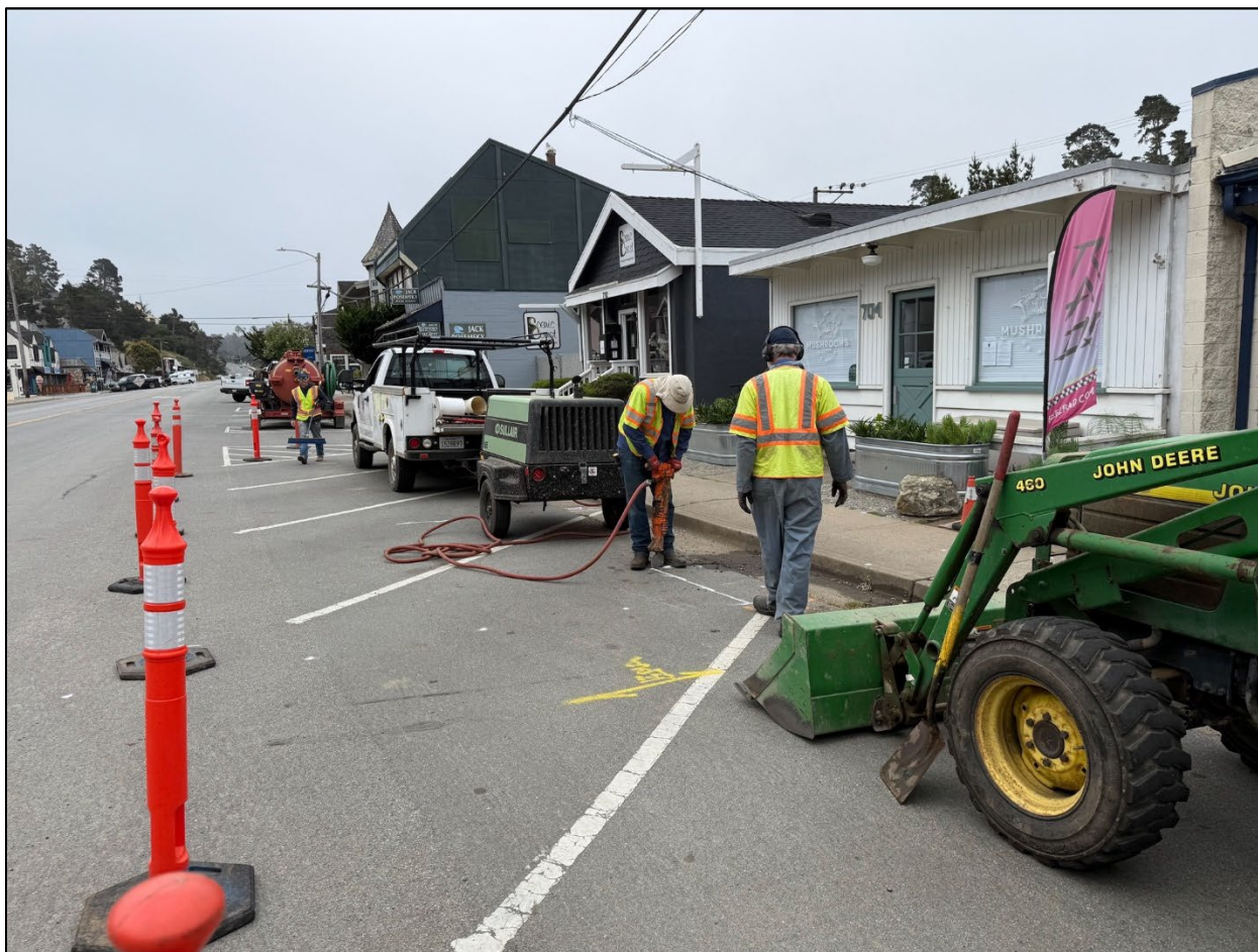
Figure 12: Start of excavation on Main Street to repair leak
