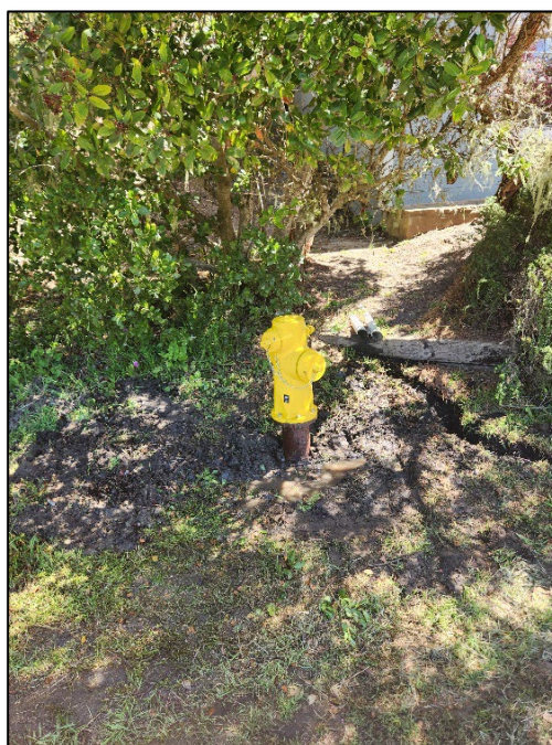
Figure 19: New hydrant with repositioning
