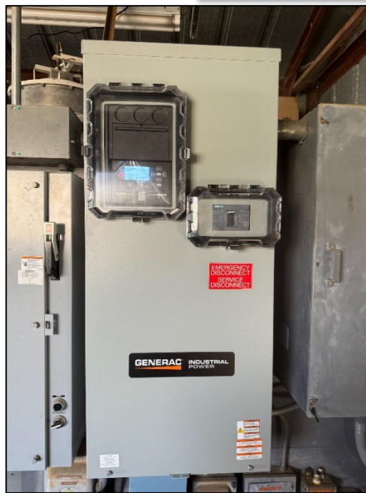
Figure 8: Newly installed Automatic Transfer Switch
