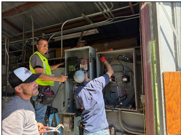
Figure 7: Work in progress to replace manual transfer switch
