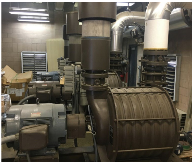
Figure 13: Existing Multi-stage blowers
