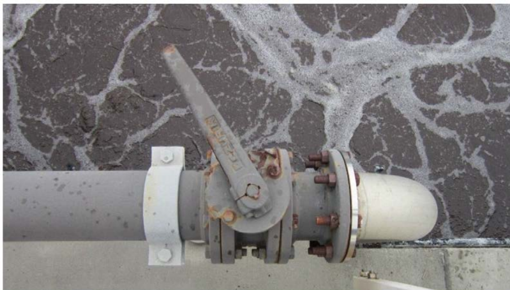
Figure 14: Partially Closed Blower Air Distribution Valve
