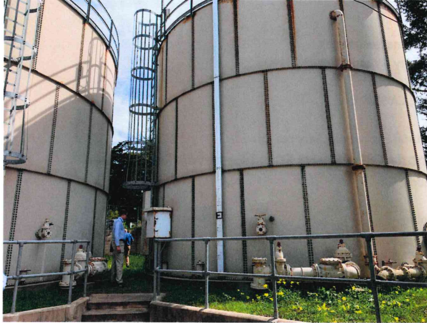
Photo of Existing Bolted Tanks to be replaced - MKN
