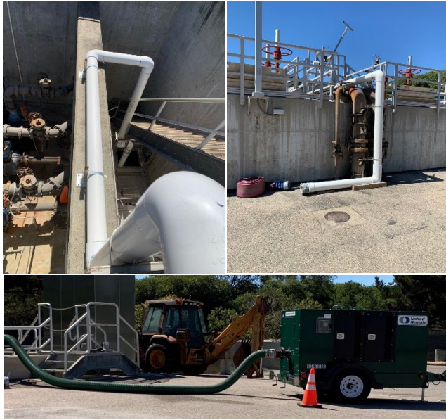
Figure A - Bypass piping from the influent wet well to the aeration basins (top) and the 6-inch pump purchased in 2017 (bottom)
