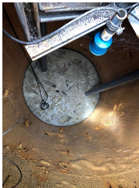
Figure C - Fats, Oils, and Grease collect in the system and cause problems by blocking lines and gumming up pumps.
