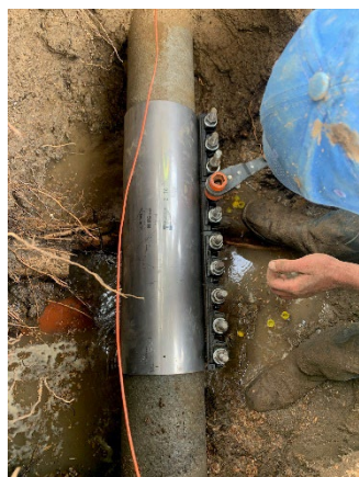
Figure D - Repair of 6" main on Lancaster
