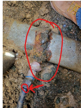
Figure E - Corroded saddle and failed service line at Burton Dr near Ardath
