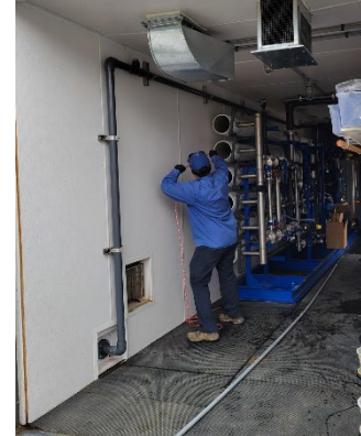
Figure F - Operator Cody Meeks cleaning vessels prior to RO membrane installation
